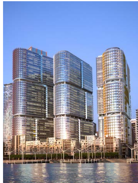
Figure 5_ IT Towers, Barangaroo by RSHP
