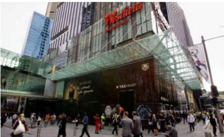
Figure 2_ Westfield Shopping Centre, Pitt Street Mall
